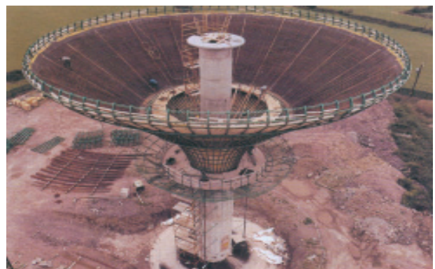
Reservoir waterproofing
