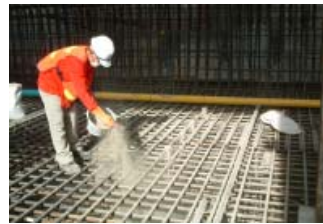
Dry shake to lean concrete
