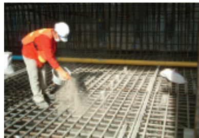
Dry shake to lean concrete
