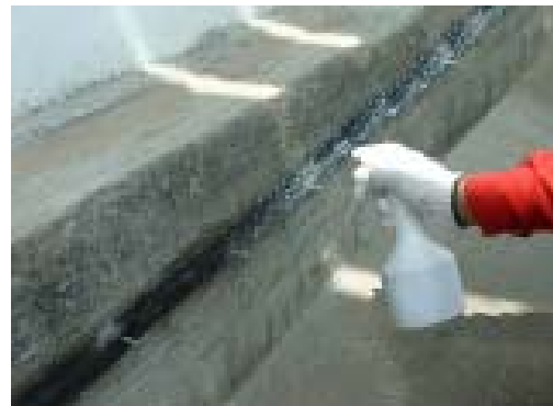
Contite Waterstop Delay Coating application by spray
