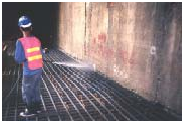
Surface preparation/cleaning by water blasting
