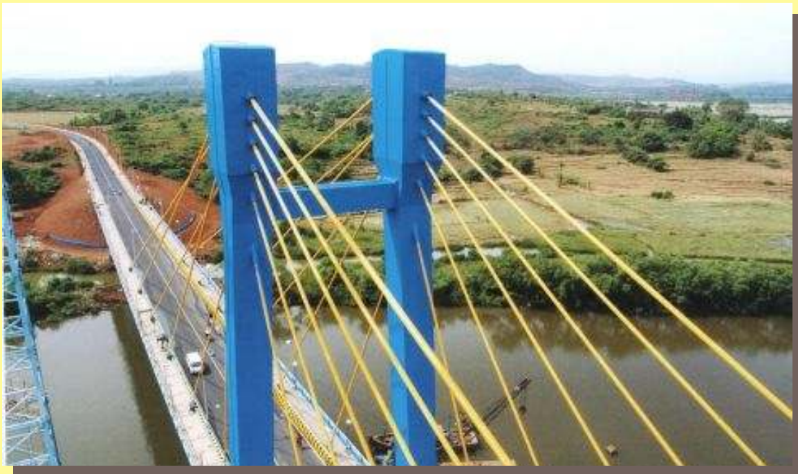
Expansion Joint Application at Cable Stayed Bridge, Goa
