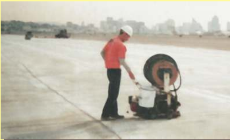
▲ Delastic® Pavement seal application with auto-installer
