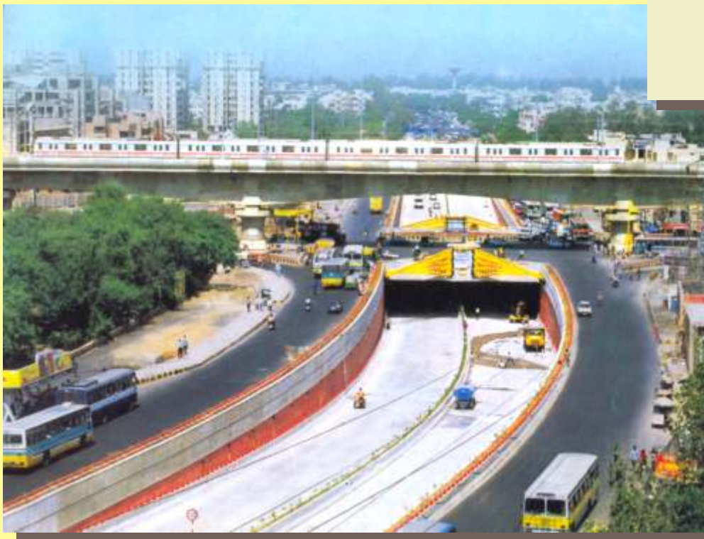
Pavement Seal Application Madhuban Chowk Flyover
