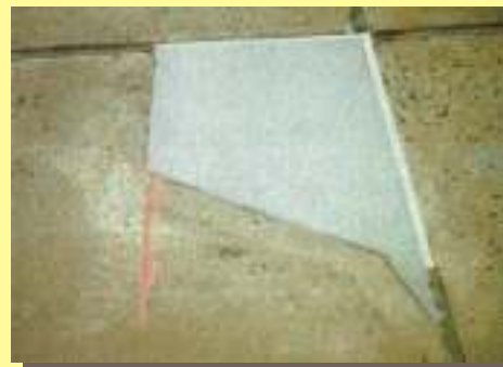
Delpatch™ Elastomeric Concrete can be used to cast airfield pavement lighting and to repair high-traffic pavement such as airport runways, taxiways and aprons.
