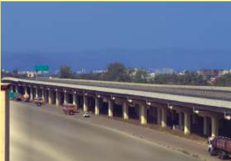
◀ Kalamboli Bridge - New Mumbai Steelfex expansion joint application
